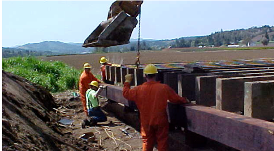
Maintenance - Bulkhead and Deck Replacement
