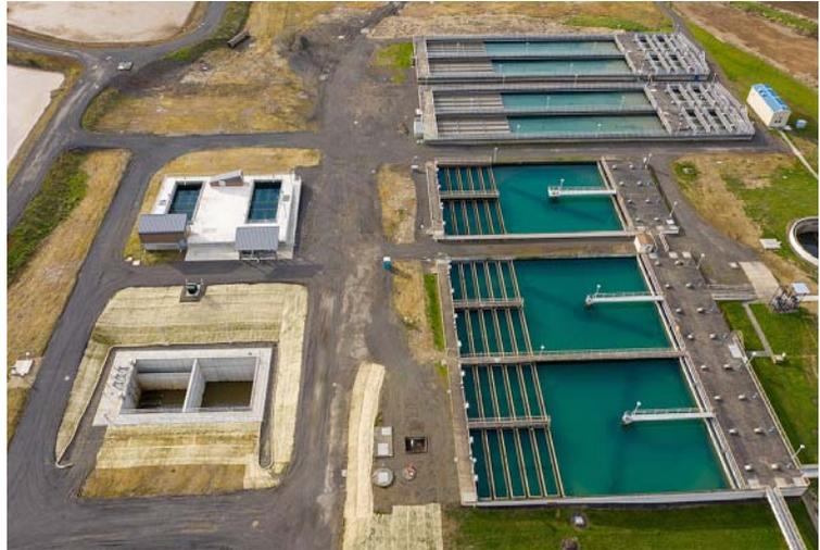
New filters (top left) and surge basin (bottom left) were constructed near the existing sedimentation basins at the JWC water treatment plant to expand capacity from 75 to 85 MGD.
