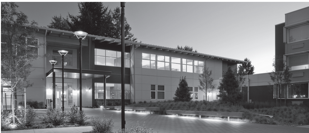
Combining CDBG, HOME, and other leveraged resources, Sequoia Mental Health Services Clinical Office Building, with Neighboring Spruce Place Apartments, providing permanent supportive housing to persons with severe and persistent mental illness
