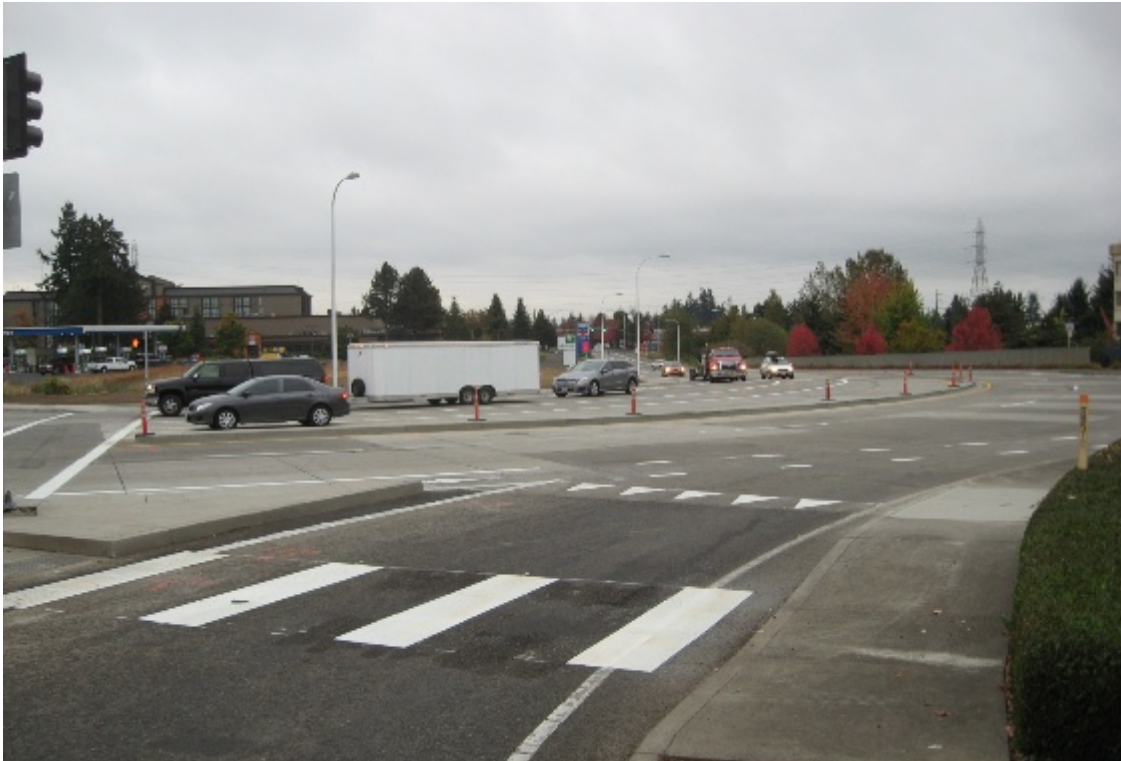
The Transportation Development Tax helped fund capacity improvements at the SW Boones Ferry Road / 95 th Avenue / Commerce Circle intersection in Wilsonville. Image: City of Wilsonville
