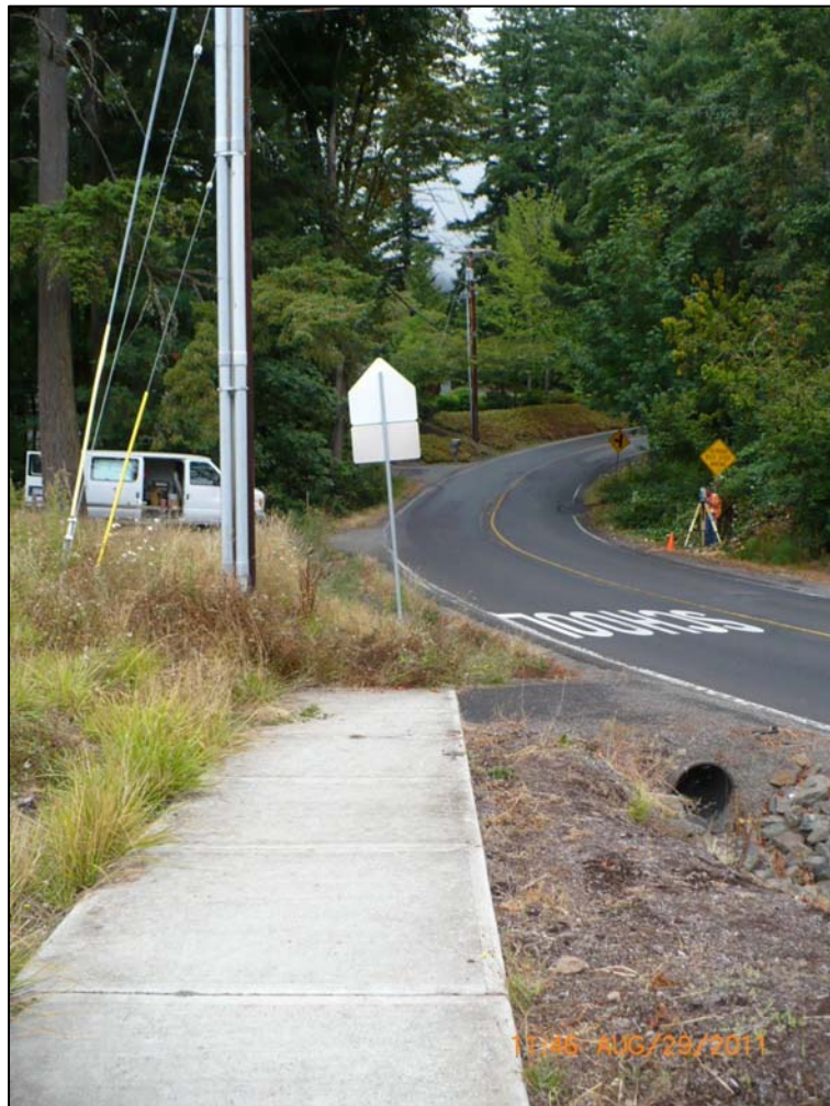
Laidlaw Road at 140th Avenue looking east
