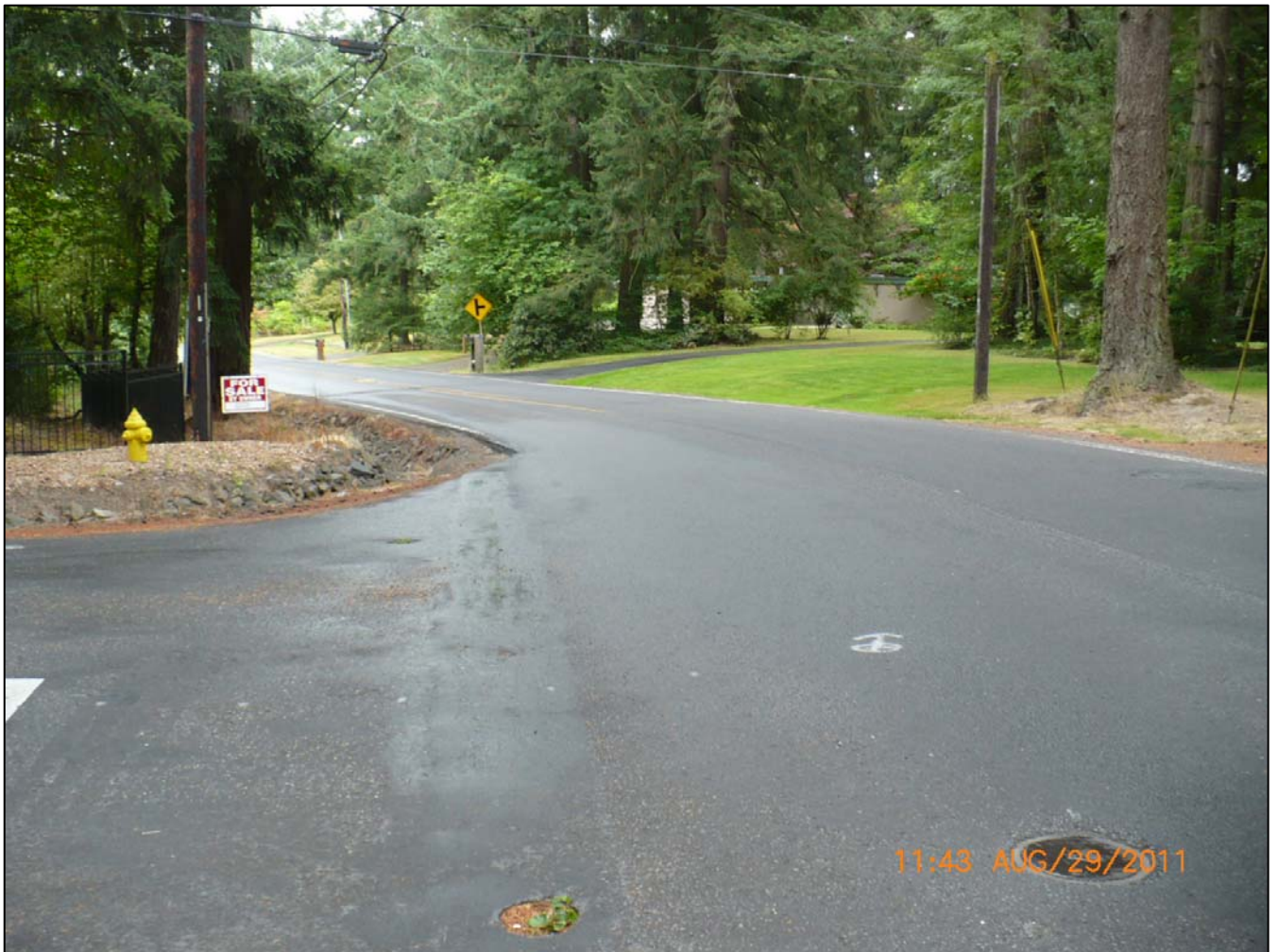
Laidlaw Road at 137th Avenue looking east
