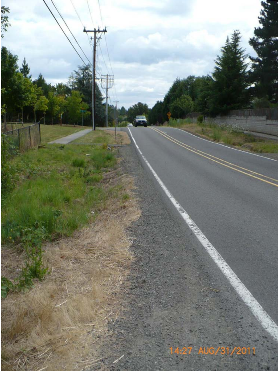
Proposed paved pathway location, east side of Kaiser Road at house #4190 facing south
