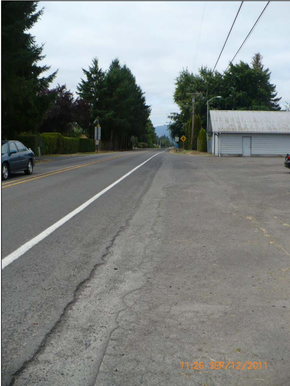
Verboort Road near Visitation Road looking west
