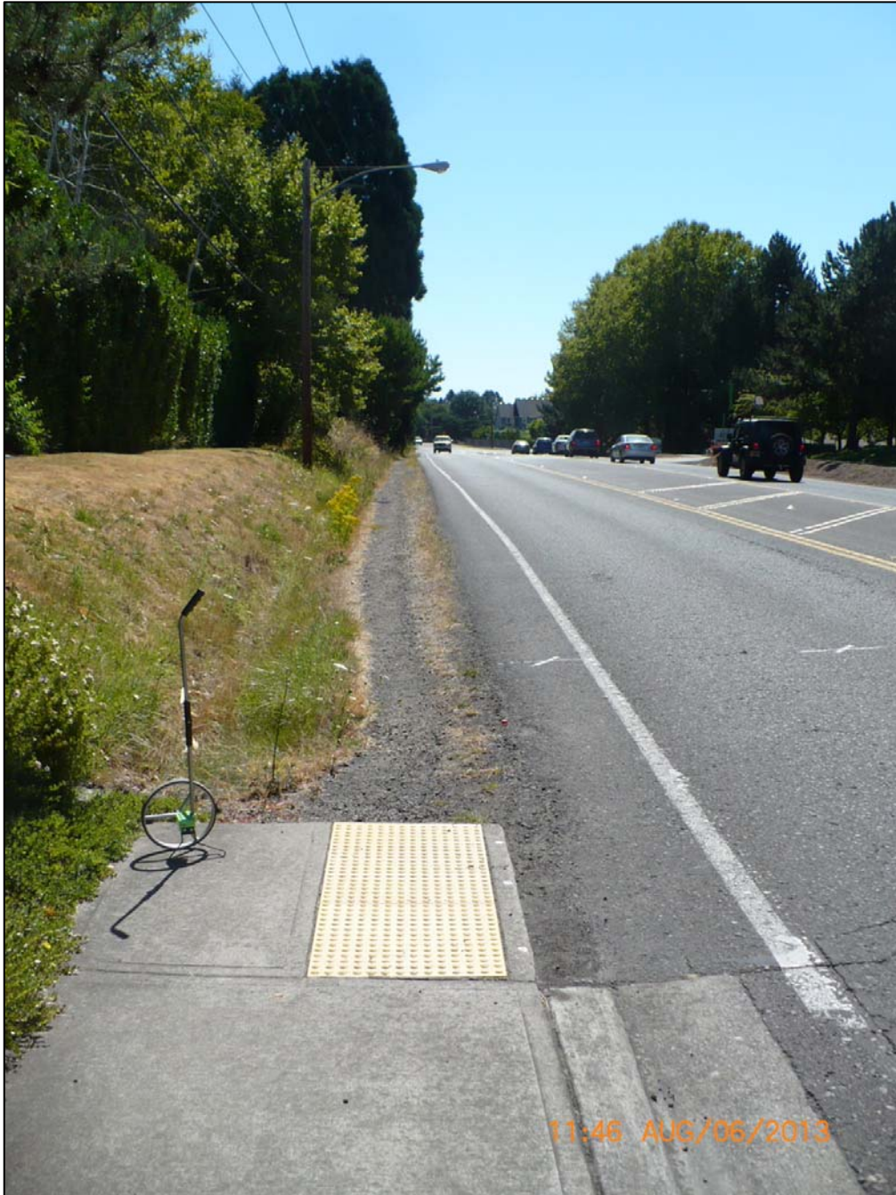
Walker Road at 183rd Avenue looking east
