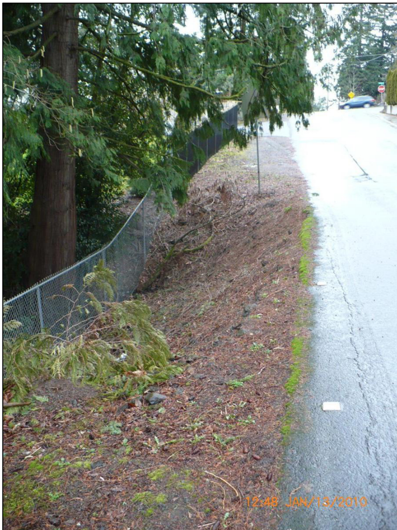
Lost Park Drive looking west
