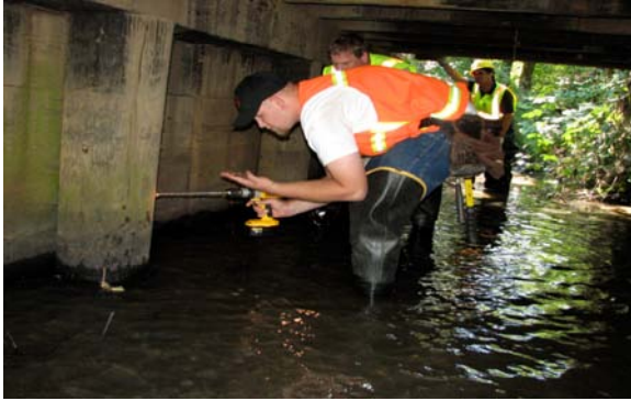
Pile Inspection – Looking for rotted wood
