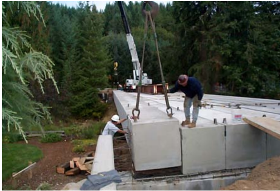
New Construction - Placement of Pre-Stressed Concrete Box Beam
