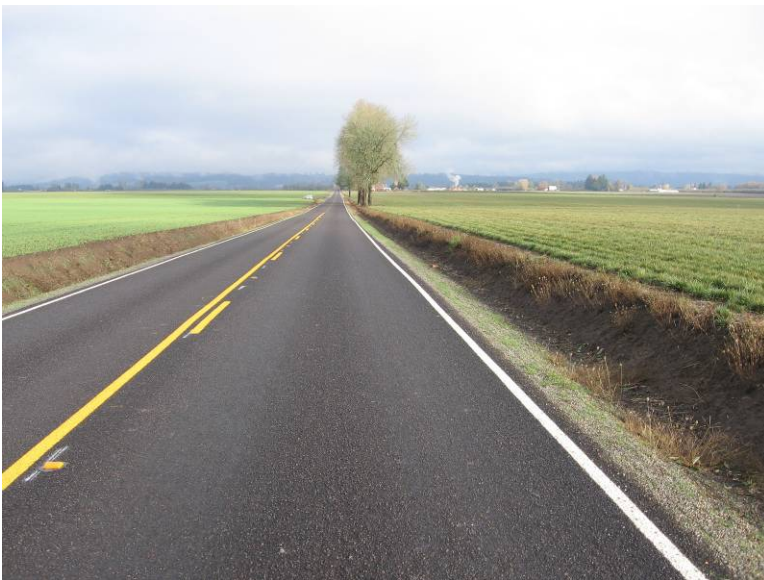
High quality chip seal on Gordon Road. Constructed in the summer of 2009.
