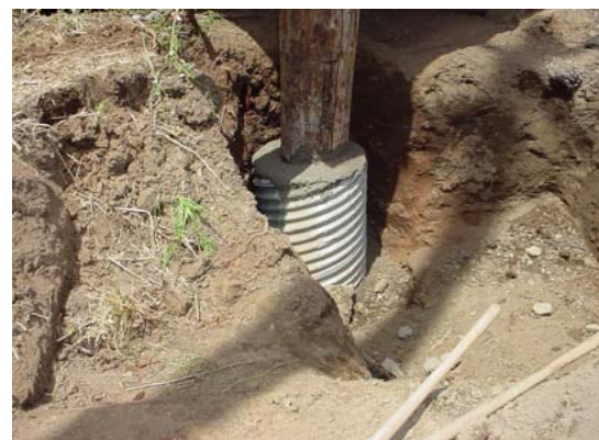
Roy Road (pile splice)
