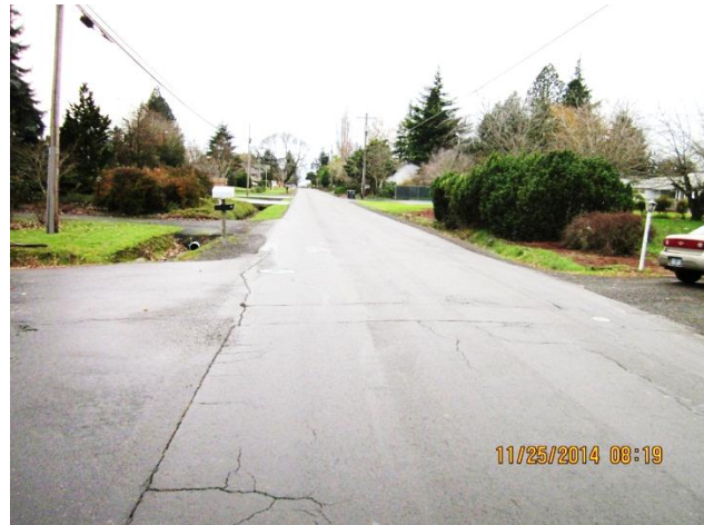
Near 200 th Ave, looking west.
