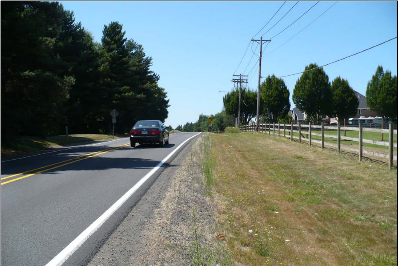
Thompson Road near Circle A Drive looking west
