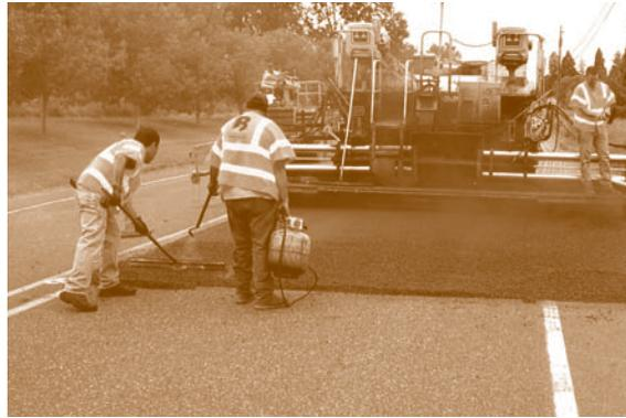
Preventive sealing of road surfaces maximizes their useful life and saves tax dollars over the long term. One dollar spent on road maintenance typically saves five dollars on future rehabilitation costs. Sealing methods vary depending on the road's characteristics:
